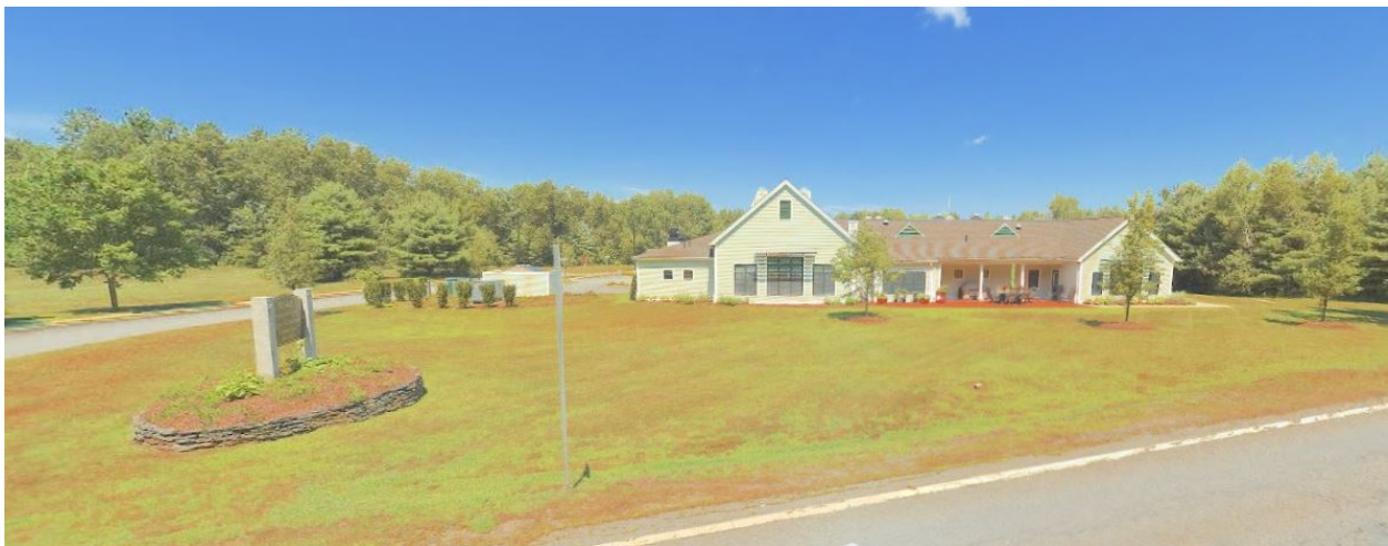
View of Erving Senior Center from Route 63. Subject Property is located out of view, behind the Senior Center.
