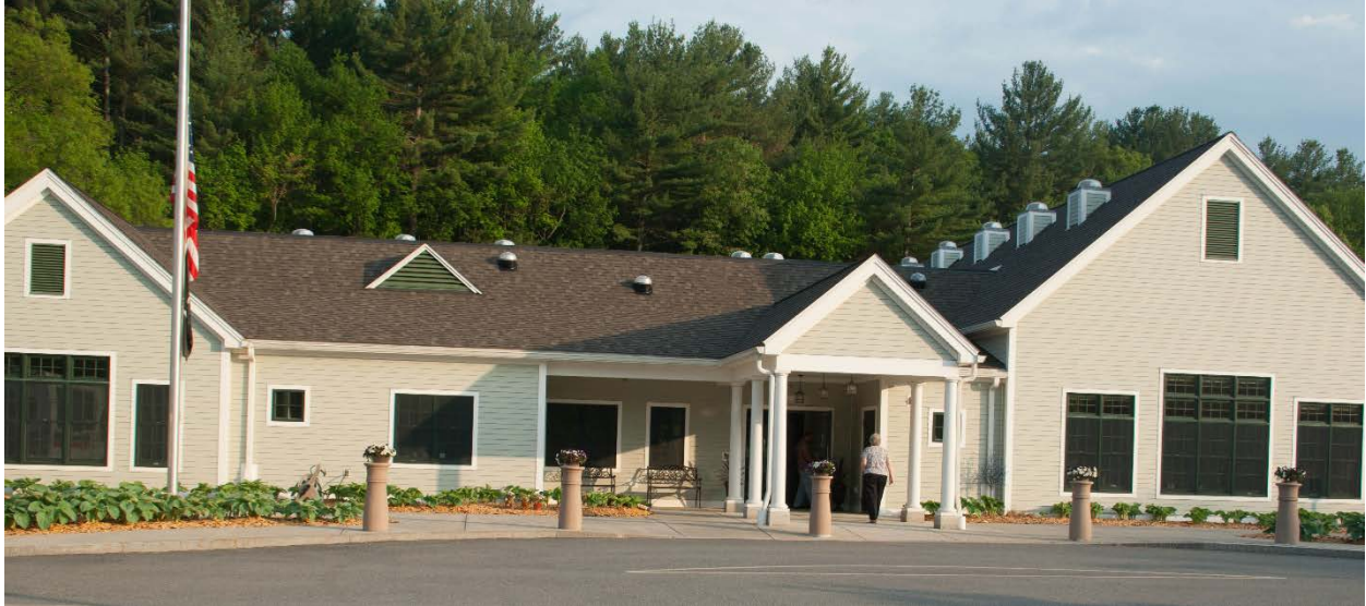
Front of Erving Senior Center, with parking lot in foreground
