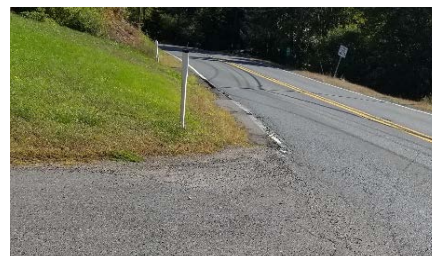
Image 5: Faded Shoulder Markings East of Wheelock Street
