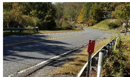
Image 1: Route 2 Approaching Holmes Avenue from Wheelock Street
