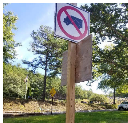
Image 16: Temporary Sign Assembly for Truck Restrictions on Mountain Road
