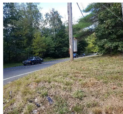
Image 17: Limited Sight Distance when Looking West from the Stop Bar on Mountain Road
