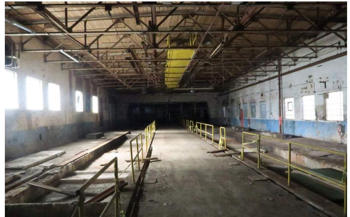
High windowsills that would need to be lowered, combined with a rotted roof structure make this wing unattractive for restoration within a reasonable budget.
