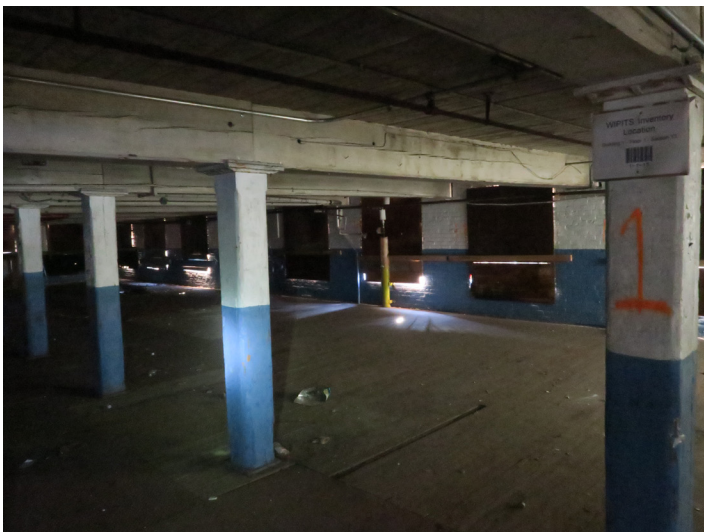
Low ceiling height on the first floor of Building 2 requires a 2-story type residential apartments with partial floor removal.
