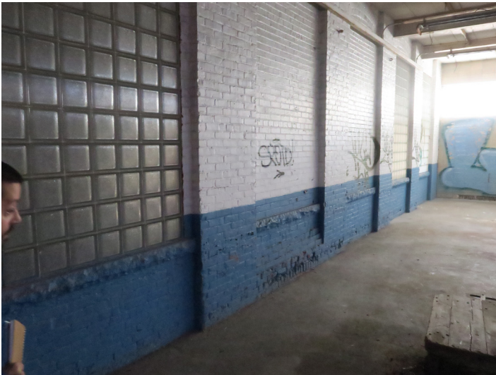
The brick work requires significant repointing in addition to paint removal.
