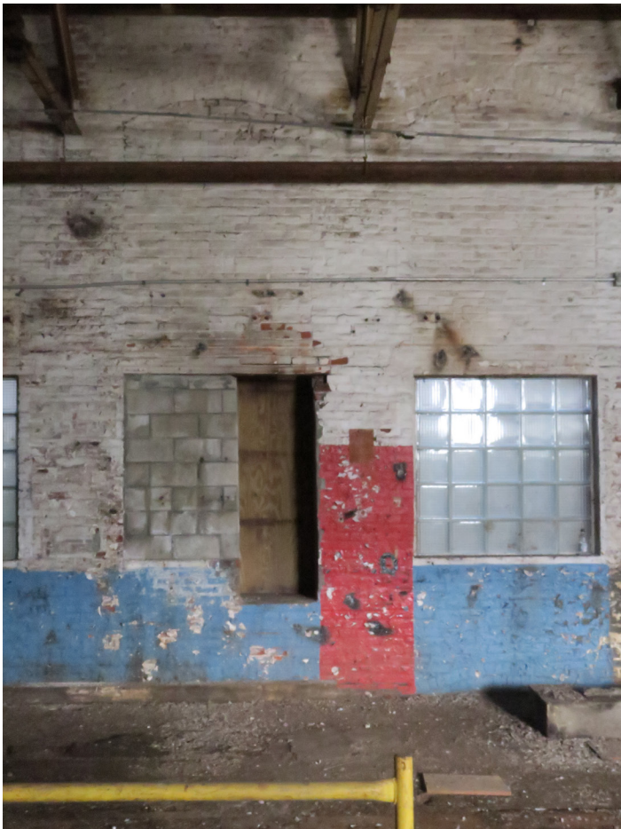
The extensive area of repair, replacement, or removal do not need to be all uniform. The "patchwork quilt" approach of the existing walls leads to an interesting surface treatment.
