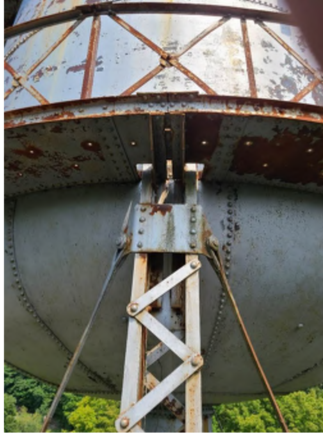
Photo 2: Typical leg connection to tower bowl
