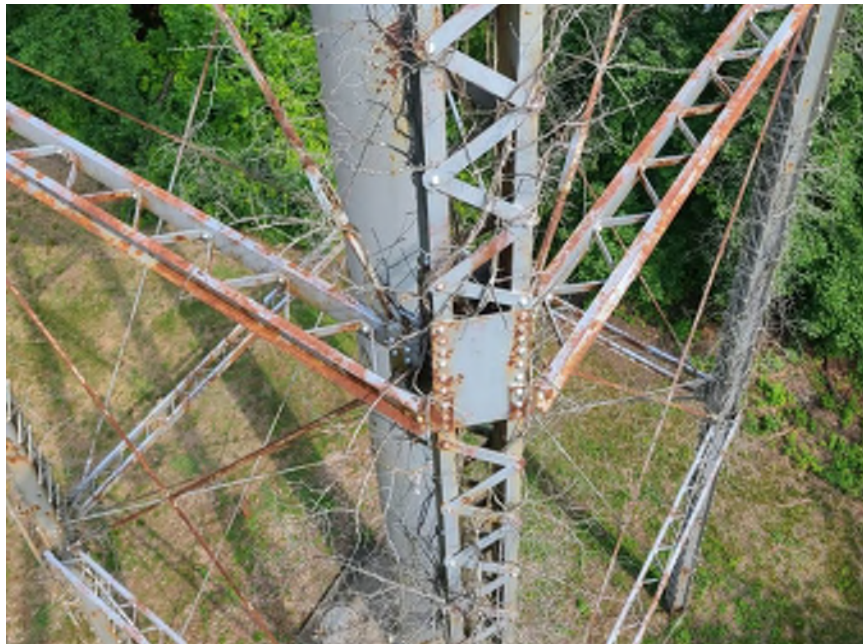
Photo 3: Typical column brace connection at column base
