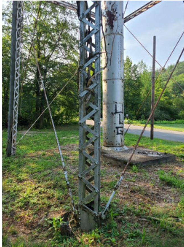
Photo 4: Typical brace to leg connections
