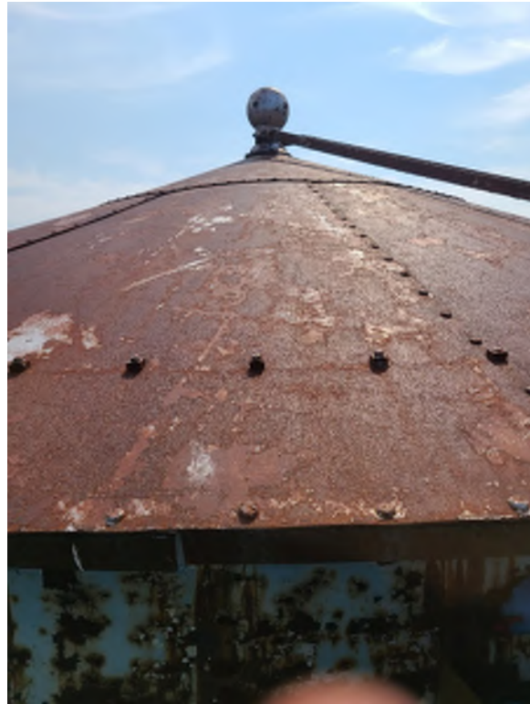
Photo 6: Typical tank roof surface
