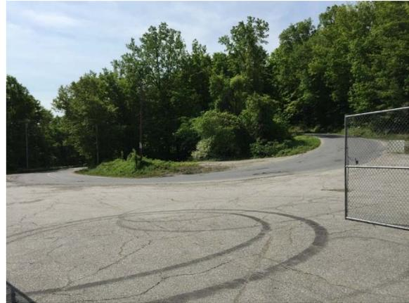
All of the concepts include a defined 24-foot wide entrance to the site located at the midpoint of the curve in Paper Mill Road to maximize the site distance to the north and south from the new entrance. Although there are no sidewalks on Papermill Road, sidewalks are proposed extending north and south from the entrance to provide pedestrian access along the sharpest portions of the curve in the road. The photo below provides a view to the west at the approximate location of the new entrance.
