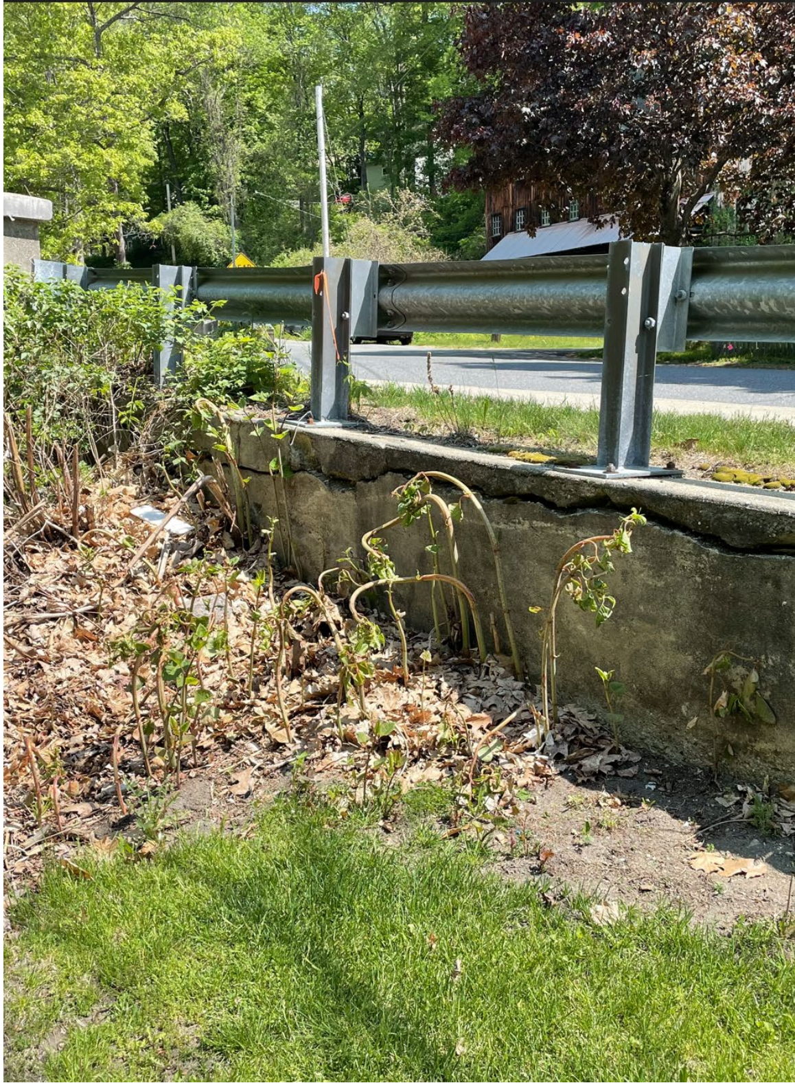
Guardrail supported on failing retaining wall with missing anchors
