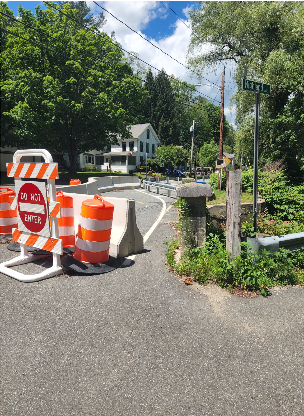
Bridge posted for 3 Ton limit with one-directional traffic
