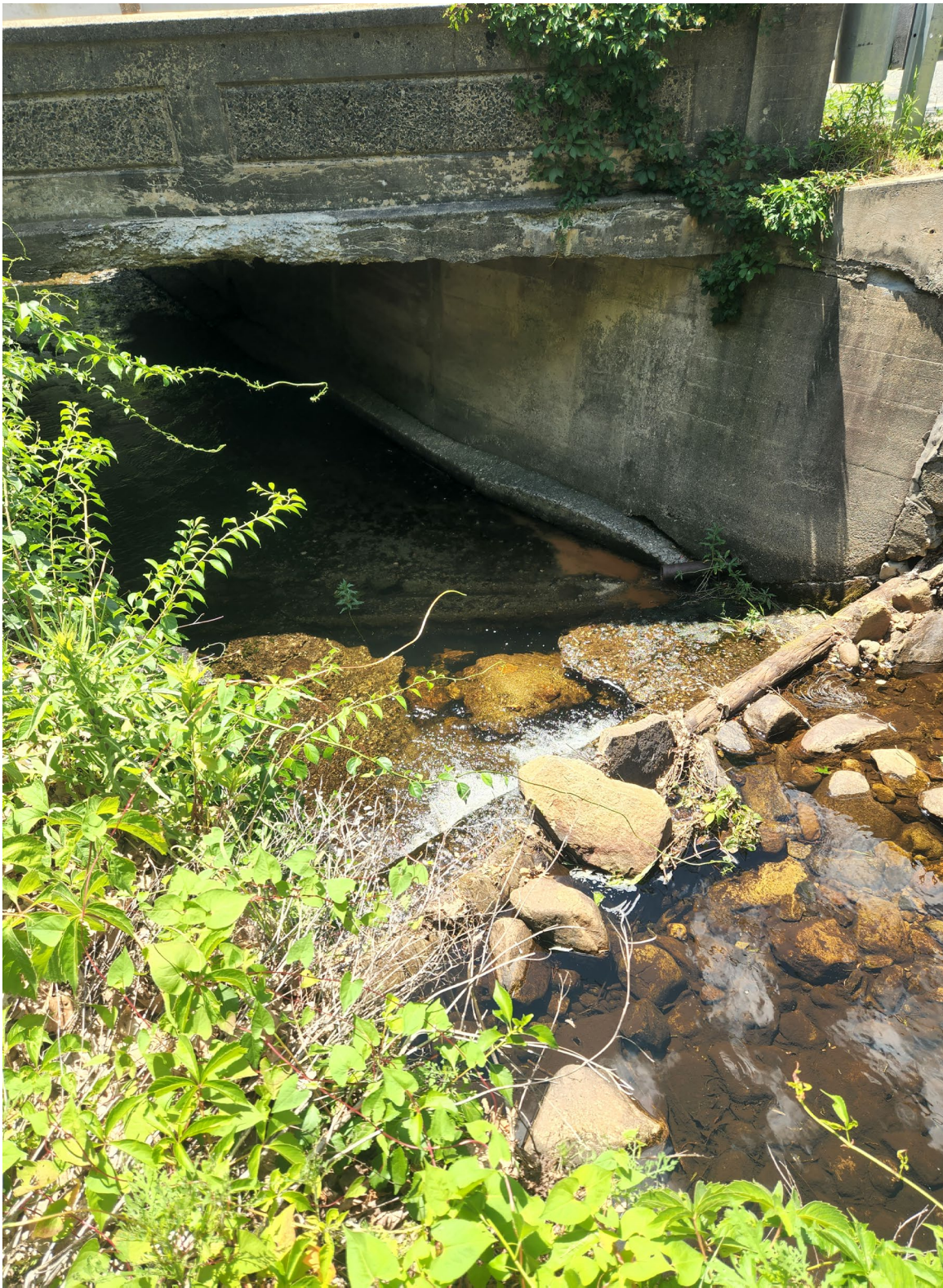
Spalling concrete superstructure
