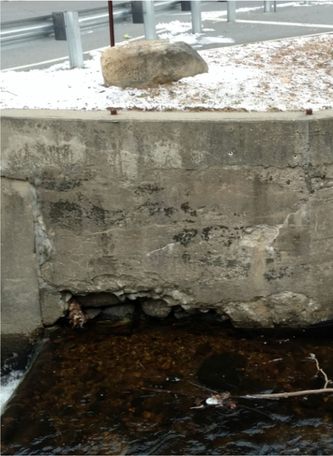
Large void in retaining wall adjacent to bridge
