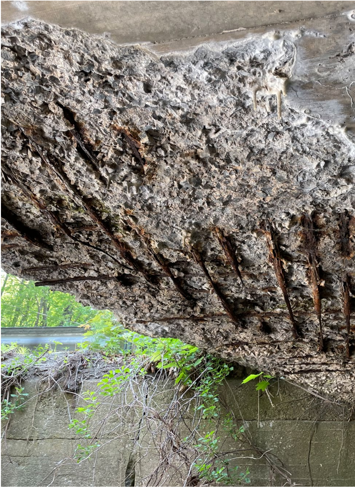
Large spalls with exposed reinforcing steel on deck underside
